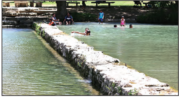
Water trickles at the Salado Creek low water dam at Stagecoach Inn. Salado Water Supply Corporation entered into outside water restrictions during the summer months due to the drought.
