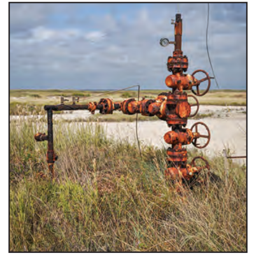
An abandoned well.
