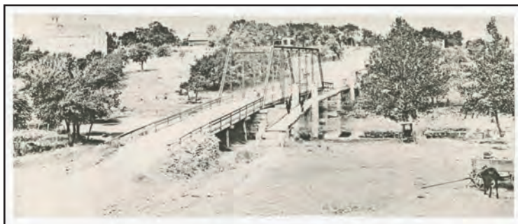
This photograph shows the first iron top wagon bridge (1892-1913) and the old foot bridge that was destroyed in 1900. (Photos courtesy Salado Historical Society)
