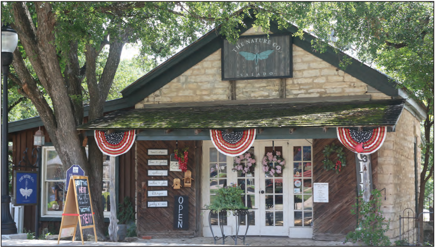
The Salado Saloon was opened for a day in this building. Today, it houses The Nature Co. of Salado. (Photo by Royce Wiggin)
