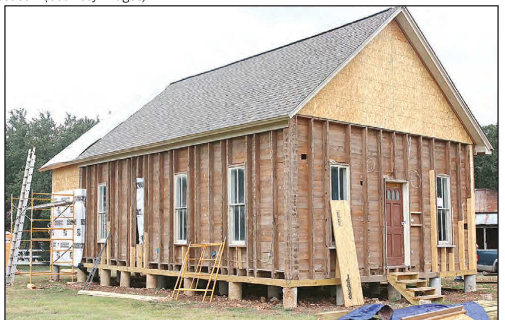
Works has begun on the 1908 Church. (PHOTO BY ROYCE WIGGIN)
