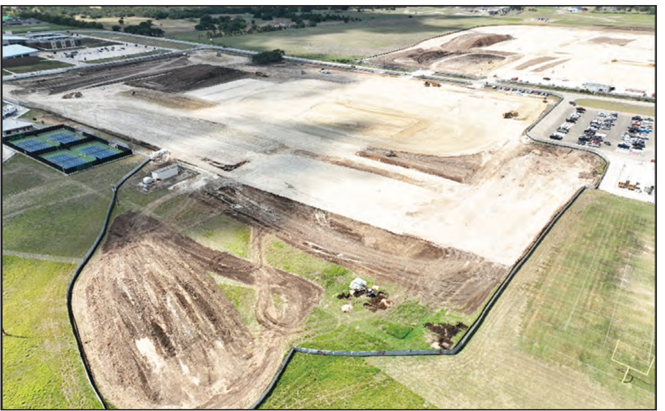
Aerial view of work at new stadium and high school.
